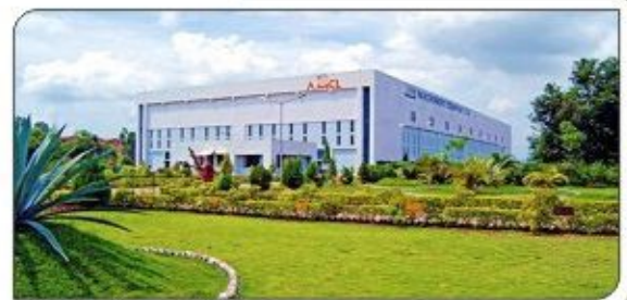
Works at Nagpur
